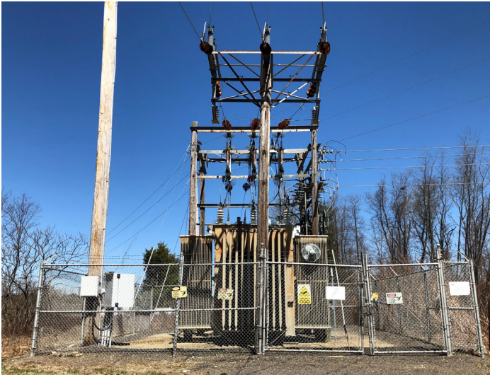
645 U.S. Route 1, Scarborough, Maine old CMP substation.
